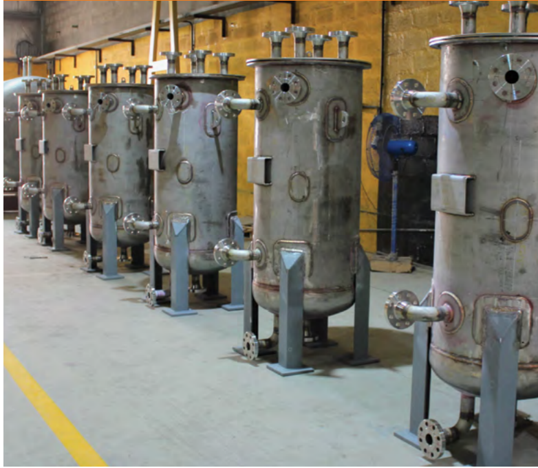
WASTE WATER TREATMENT - POLYMER DOSING STATION. End User: SAUDI KAYYAN
